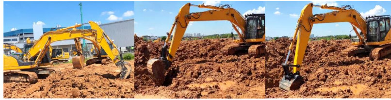
Figure 2. Excavation test process.
