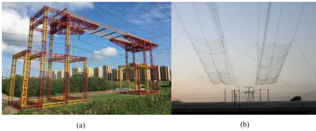
Figure 1. Two different forms of cross frames: (a) double-gauge propulsive and (b) flexible protecting system.
